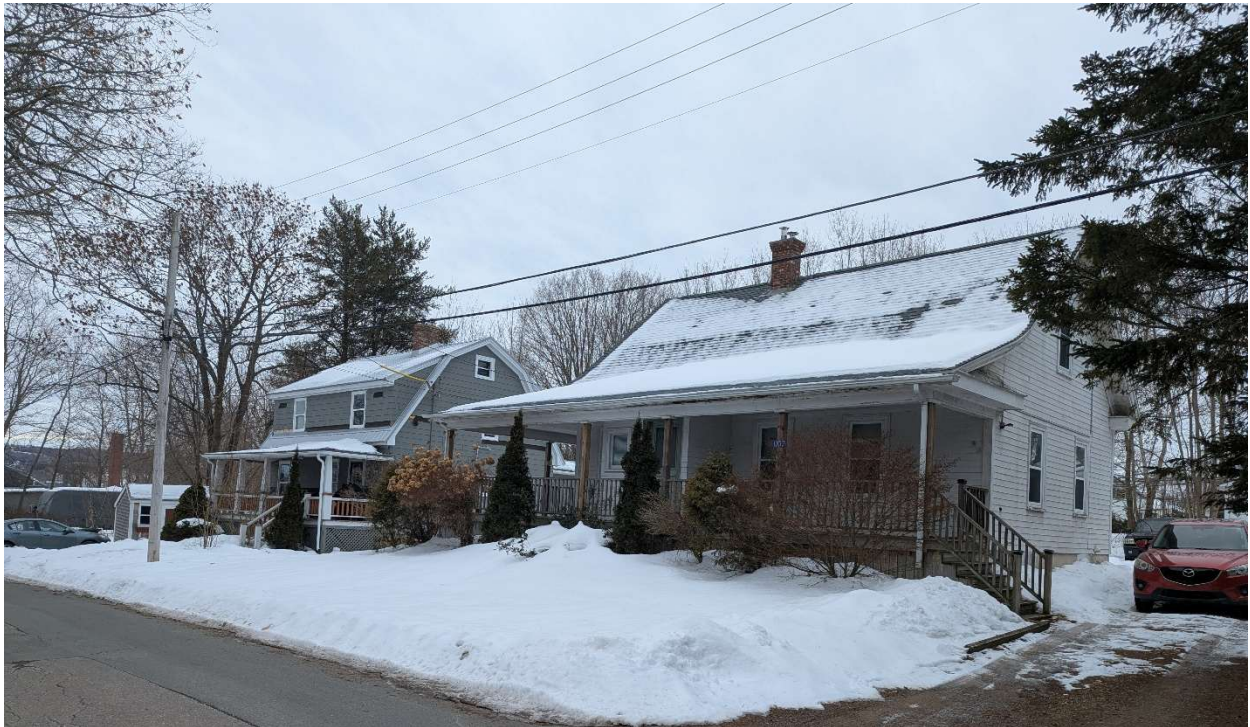
Photo 5: 1103 and 1107 Middle Street
