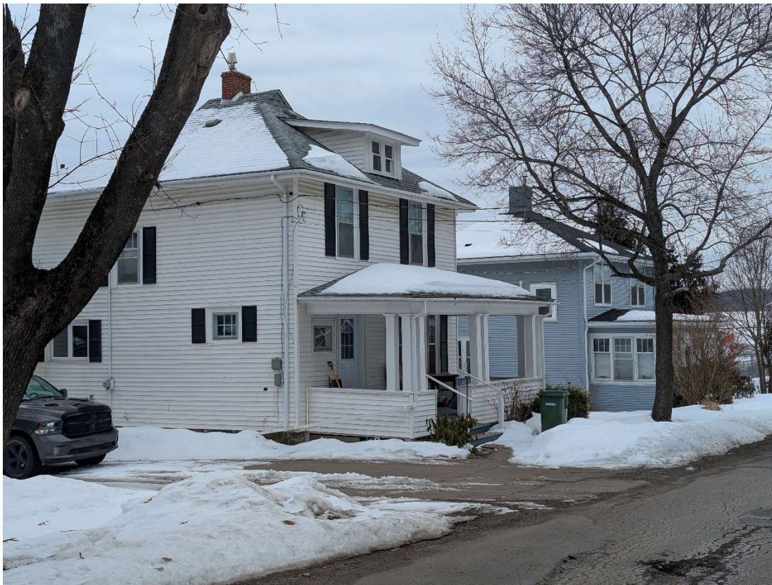
Photo 6: 1100 and 1096 Middle Street
